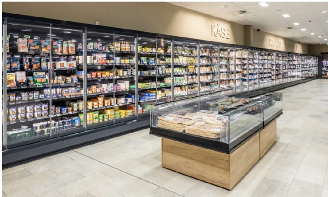
Epta's remote CO 2 -based SkyView Plus cases with doors were installed at the new Edeka Schneider supermarket in Hambach, Germany. (Source: Epta)
