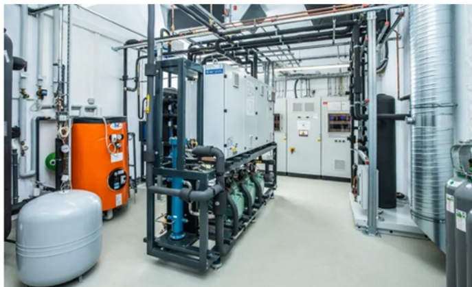
Epta's ECO2Middle refrigeration system installed at the new Edeka supermarket in Hambach, Germany. (Source: Epta)
